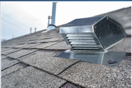
Roof Exhaust Vents
